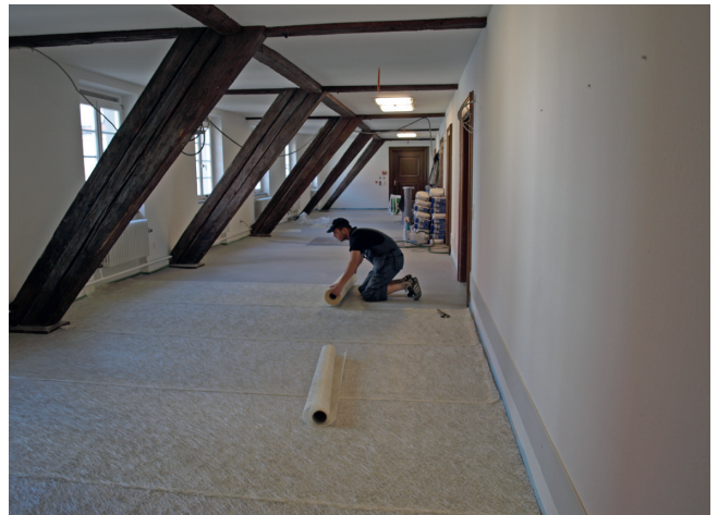
Spread UZIN RR 201 over the entire surface to be renovated.
